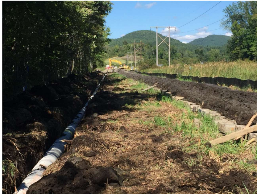
Photograph 4: Station 1649+00; trenching and lowering in the pipe through Clay Plains. Topsoil and subsoil are segregated and placed on timber mats. Photograph taken looking north.
